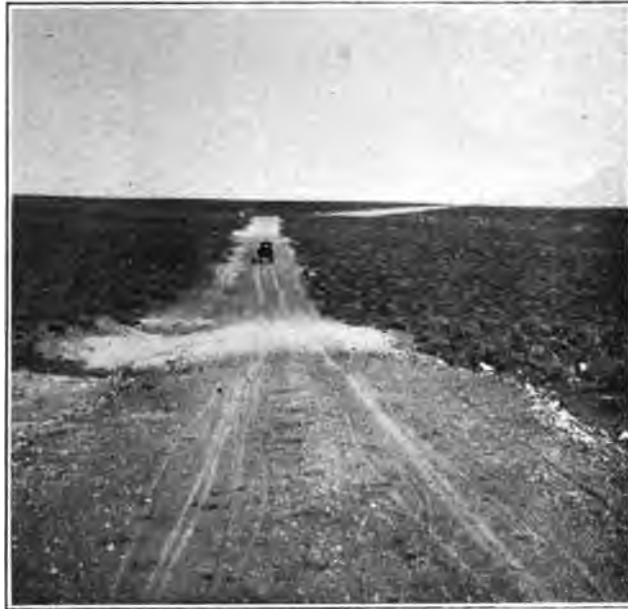
NEW STATE ROAD, PIUTE COUNTY.
